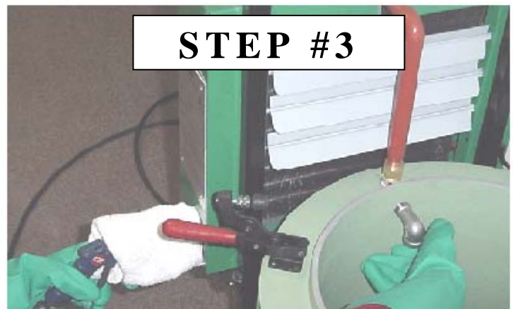
Blow air into the pipe until all objects (liquids & solids) have been ejected from the radiator.
